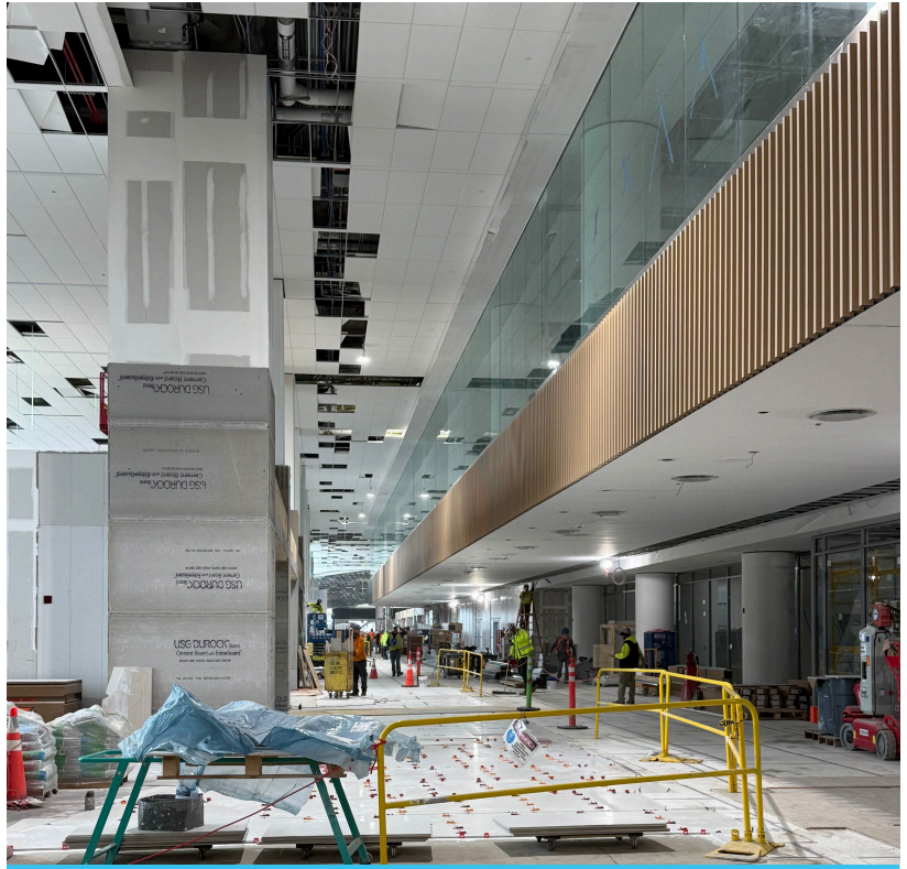
Terrazzo floor tiles being installed in concessions area
