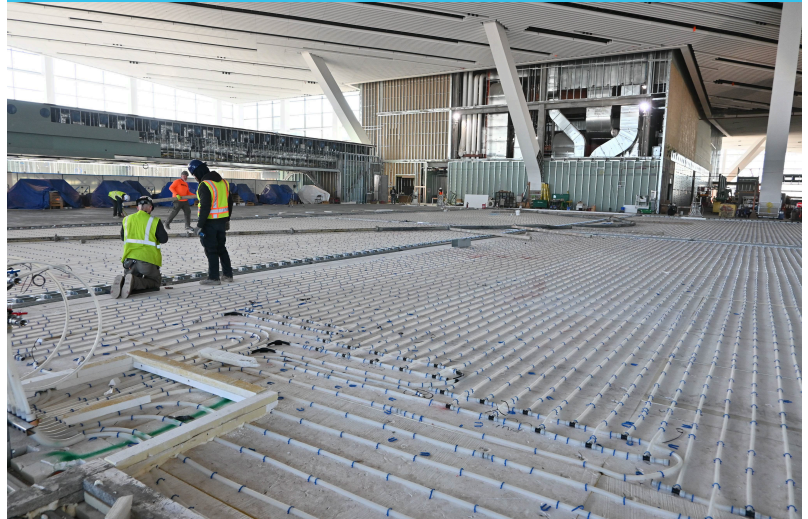
Radiant flooring being installed near check-in counters
