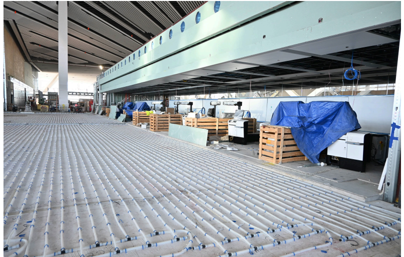
Radiant flooring being installed near check-in counters
