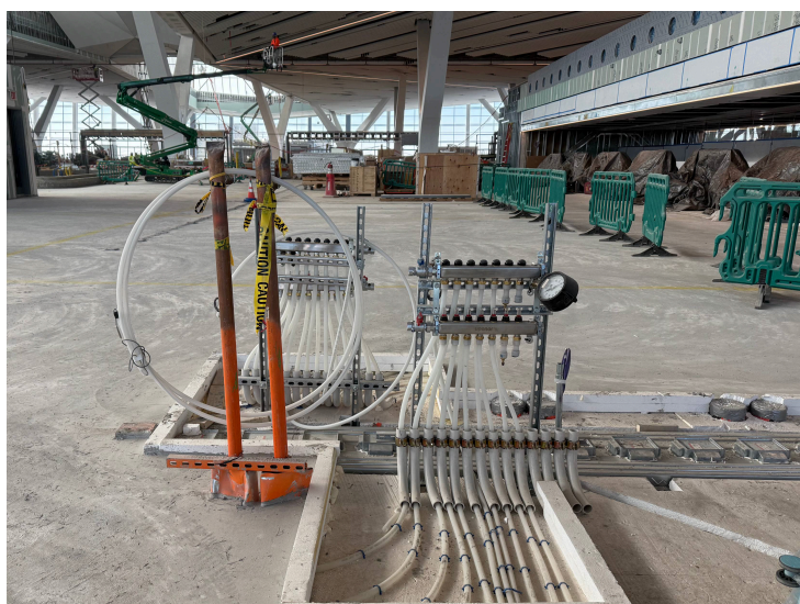
Mechanical for Radiant Floor System
