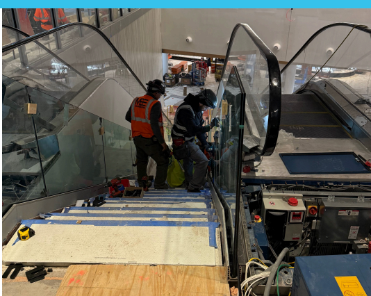
Ongoing Installation and Testing of Vertical Transportation
