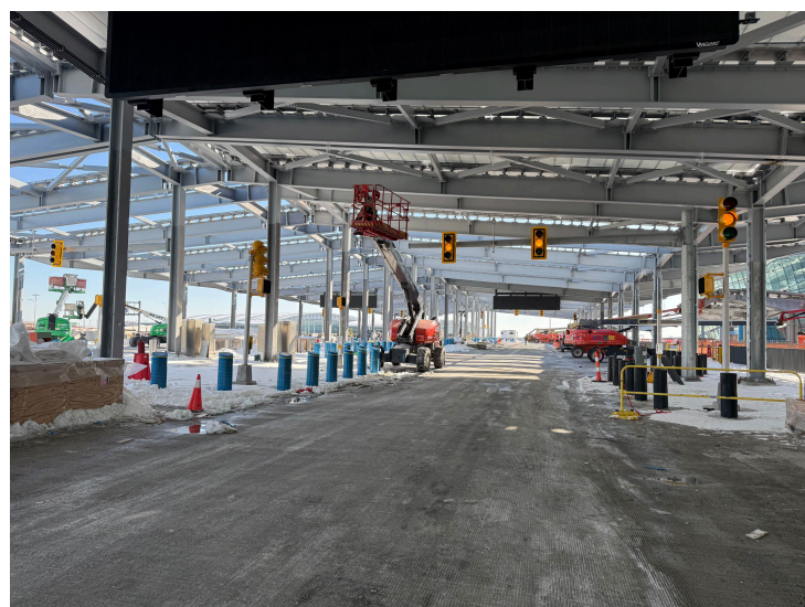
Traffic Signal Testing on Departures Level
