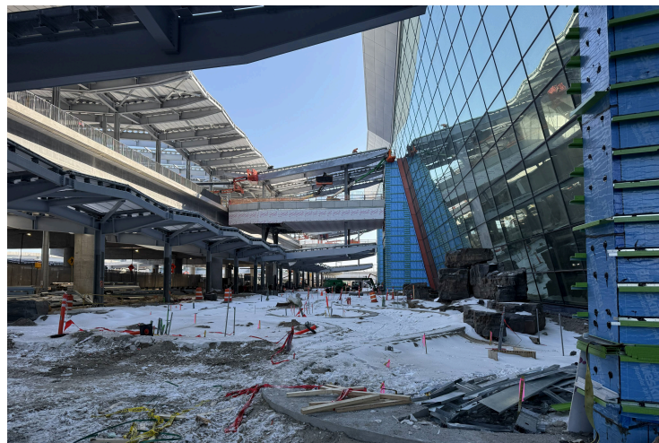
Landscaping Work Continues on Arrivals Level
