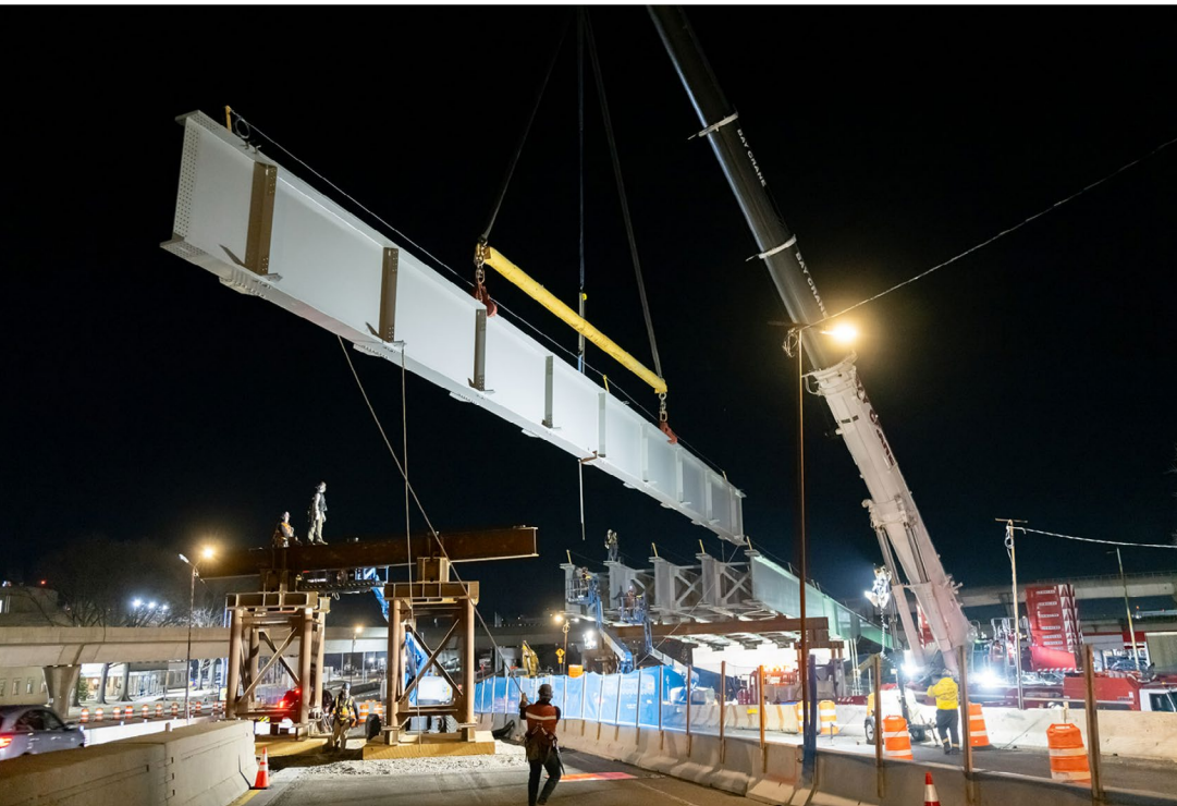
Steel Erection of J34 Steel Bridge Work, Major Event for Westbound Connector Project
