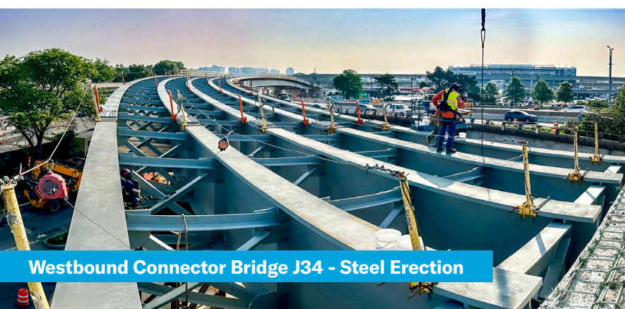
Westbound Connector Bridge J33 - Steel Erection
