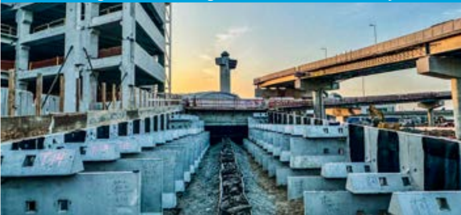
Image Left: New Garage Constuction Image Right: Terminal 4 Departures Access Bridge Foreground: New Garage Precast Concrete Assembly
