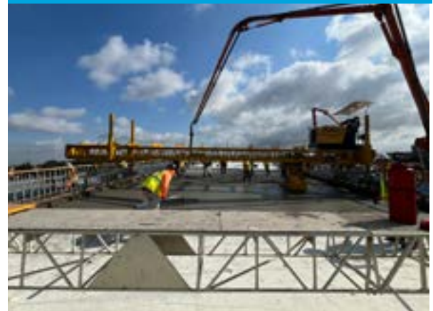
Westbound Connector - Concrete placement to finish grade for J34 roadway
