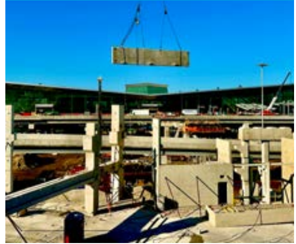
Background: New Terminal One Foreground: New Garage Precast Concrete Assembly
